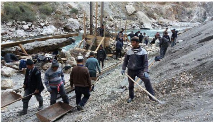
Fig. 2. Ashar in building of bridge
